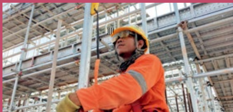
▲ Foreign staff working for the RAPID Project in Malaysia
